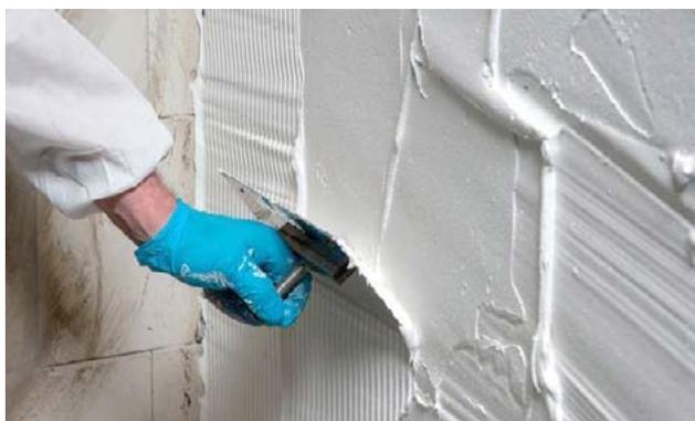
with the finishing trowel for an easier installation of the KÖSTER Glass Fiber Mesh/KÖSTER Flex Fabric reinforcement. The second coat is to be applied the same way as soon as can be done so without damaging the first coat.
